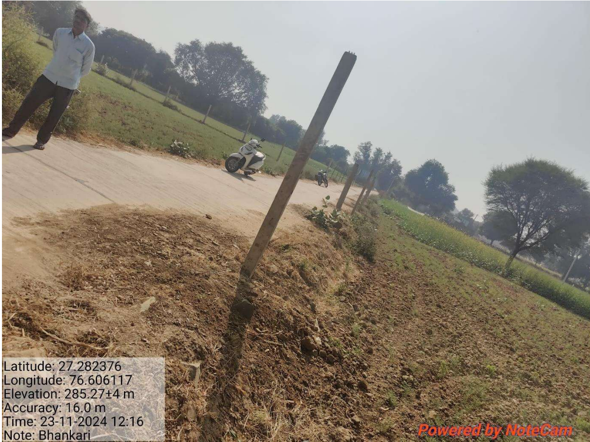
Figure 03: Newly constructed RCC road with no trees near applicant's fields where trees were uprooted
